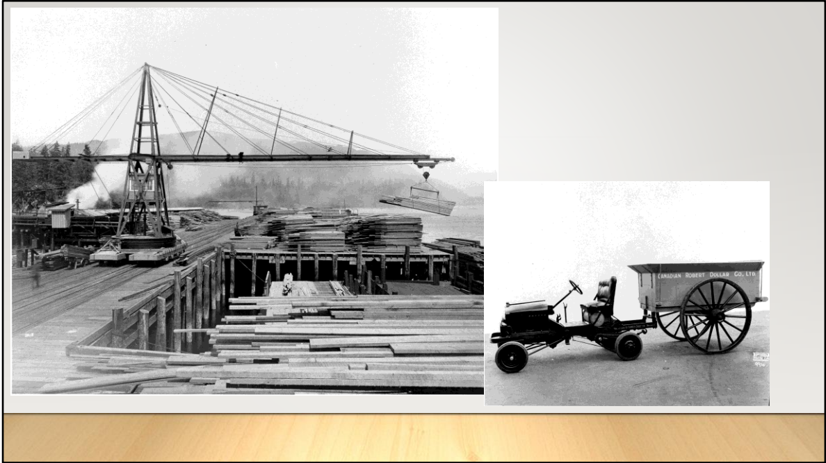
Electric crane with a load of lumber 1919 and lumber tractor and wood wagon 1918.
