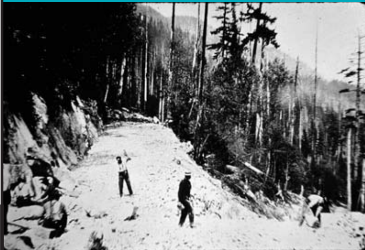
Photo #0189 - Men working on road to Woodlands c1910
