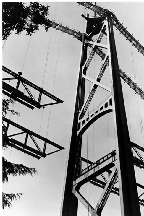
"The first section of the steel roadbed... was raised from a scow to the centre of the span by a steam hoist on shore... In twelve days 174 sections, weighing 1,572 tons, were in place." *Lions Gate*.
